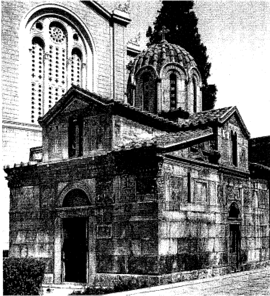
Fig. 1: Athens, church of Haghios Eleutherios, general view from the South-West (Ch. Bouras and L. Boura, Ἡ ἑλλαδική ναοδομία κατὰ τὸν 12ο αἰῶνα (Athens, 2002).
